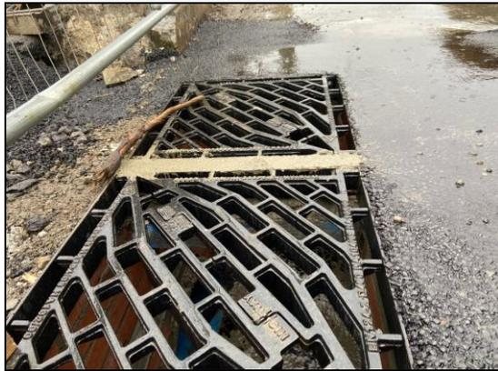
Picture above shows the newly installed storm grids outside Laxey School Gates
